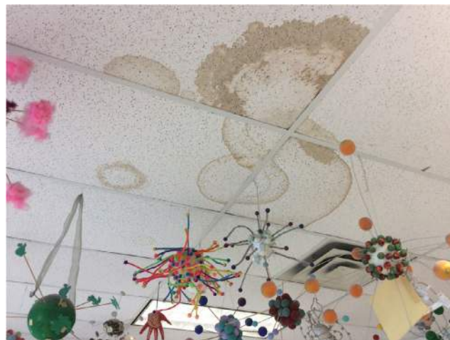
FIGURE 1 An example of visual evidence for mold growth due to water damage from water pipe leakage on a classroom ceiling. This was commonly observed at multiple schools
